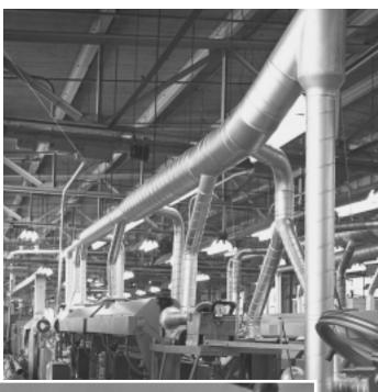
Dust control and particulate conveyance (woodworking)
