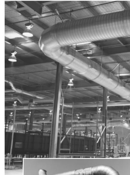
Elevated temperature exhaust (incineration)
