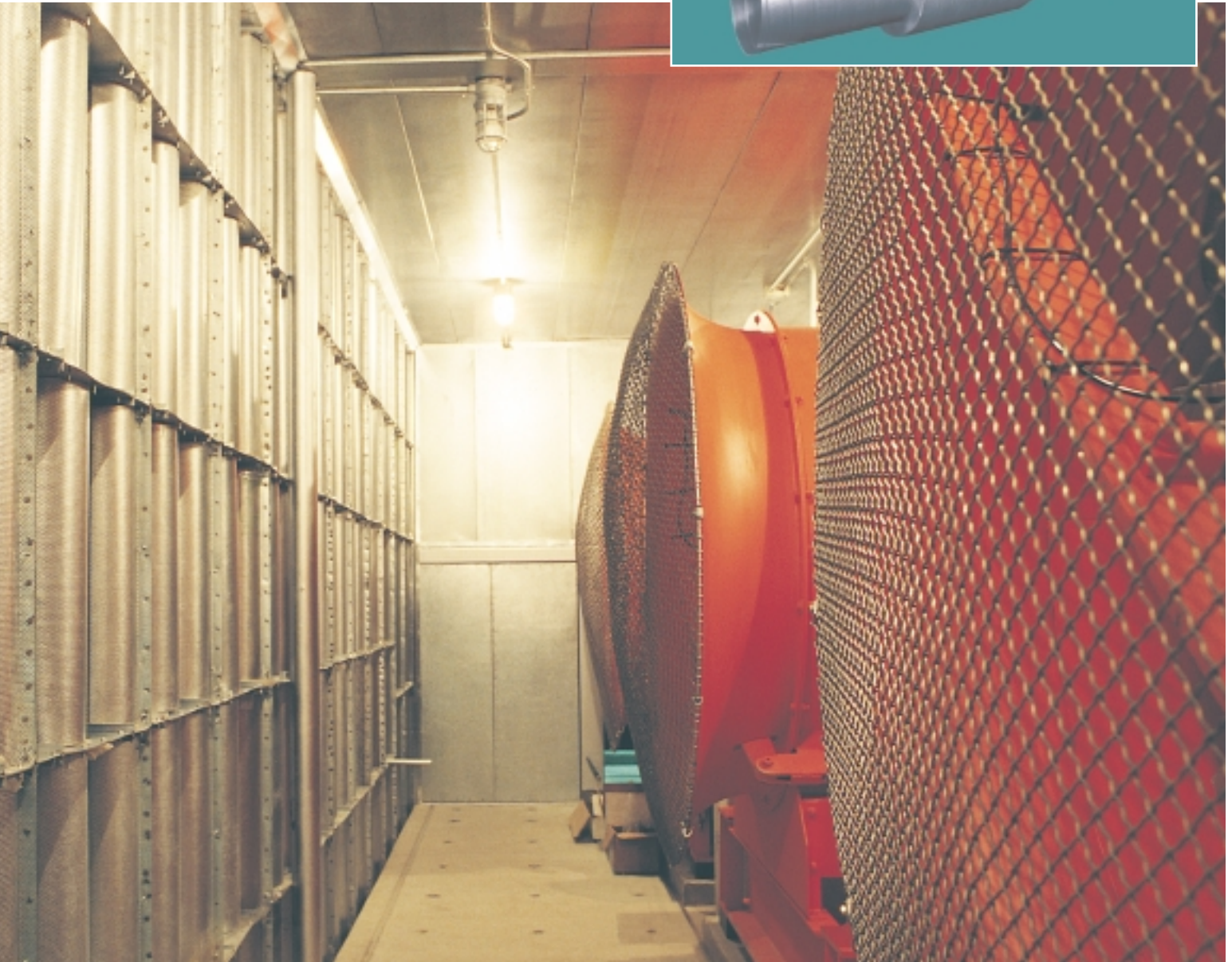
Fan Room with Rectangular Silencers, ADM—Austin, Texas
