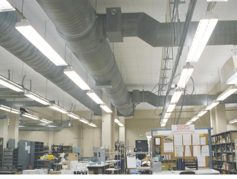
United McGill's factory-fabricated duct and fittings were a big part of the reason that the duct systems have less than 1 percent leakage.
