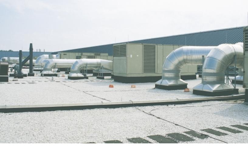
ACOUSTI-k27® double-wall, insulated ductwork is used to convey air from 28 rooftop air handling units.
