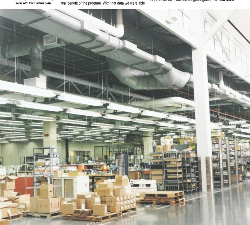
The UNI-DUCT® computer program used the static regain method to design the building's round and flat oval duct svs-
