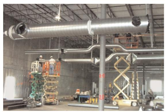
The one-percent maximum leakage allowance was also better met with spiral duct. "That variance is nearly impossible with rectangular duct," says Rick Boyer, sales manager and engineer for McGill AirFlow. "Rectangular duct requires more joints than spiral duct because it is only available in five-or six-foot sections; spiral duct is available in 20-foot sections. Each joint creates an increased possibility for leaking."
