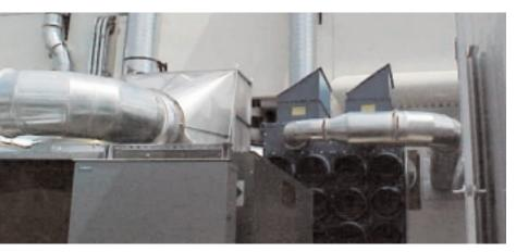
Aspire Pharmaceutical's installed HVAC system includes 6,400 feet of supply and return ductwork and 85,000 pounds of metal for the eight air handling units.
