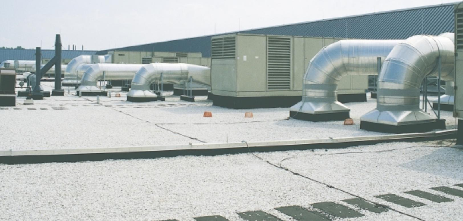
***ACOUSTI-k27® double-wall, insulated ductwork is used to convey air from 28 rooftop air handling units.***
